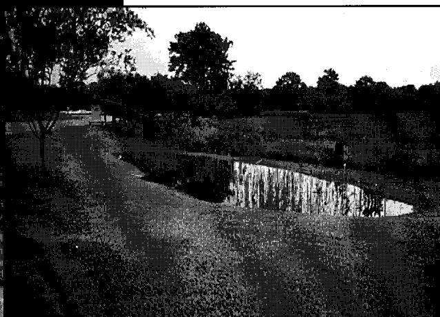
Pretreatment Sediment Basin ▲
