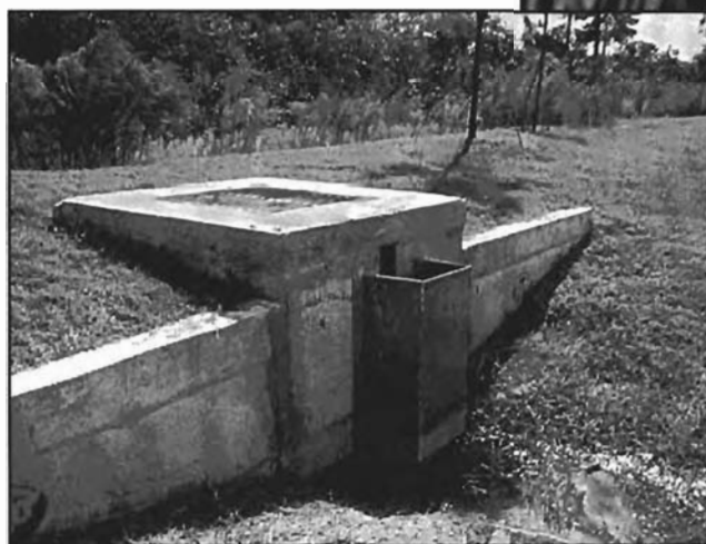
▲ Outflow Control Structure
